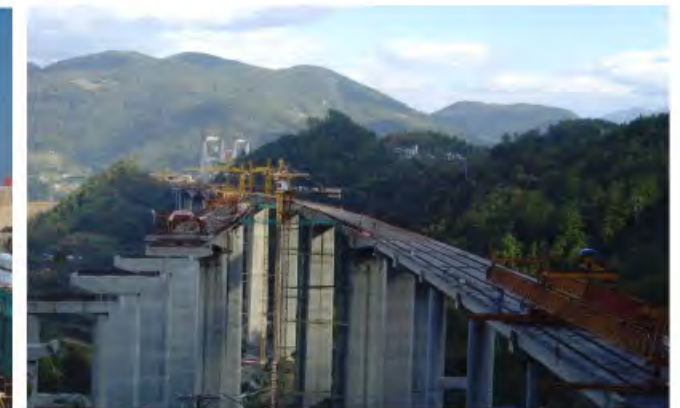
SHUINAN GRAND BRIDGE AT HURONGXI HIGHWAY, CHINA Left bridge 917.75m, right bridge 953.23m, highest pier 98m 2008 Supply and installation of PT
