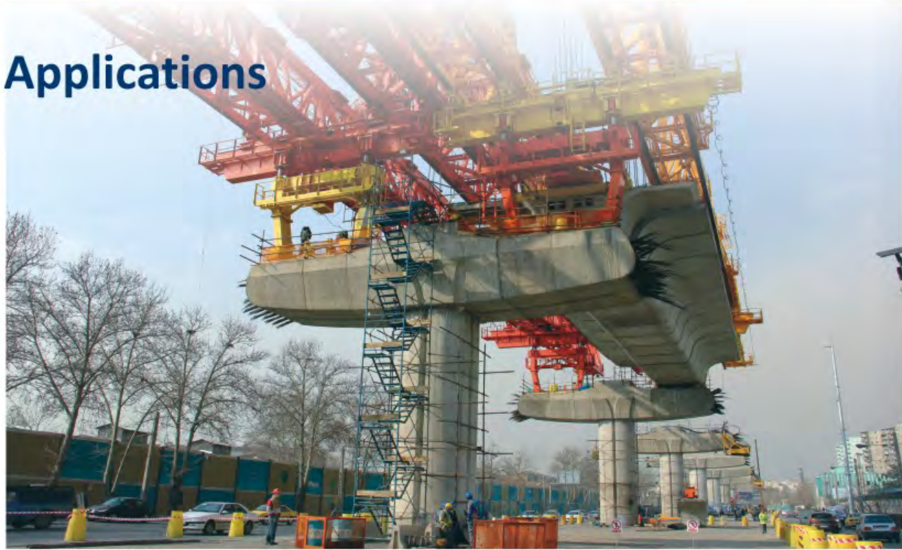
Sadr Bridge, Iran, 2012
