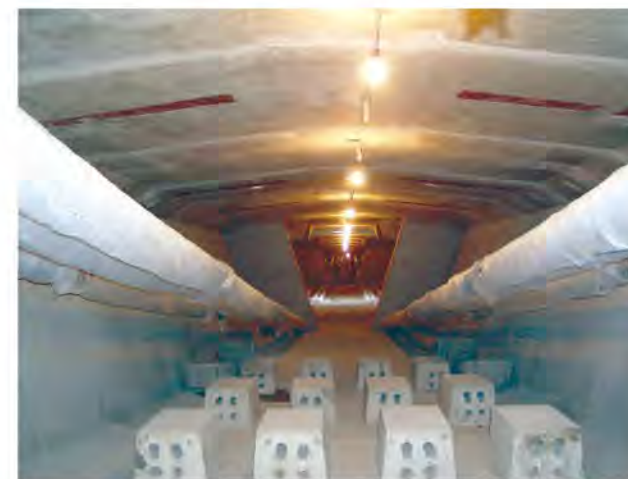
OVM External Prestressing System applied on Sutong Bridge, China
